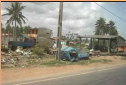
Galle – one of the worst hit areas. Houses have still not been rebuilt nearly 3 years after the disaster.
